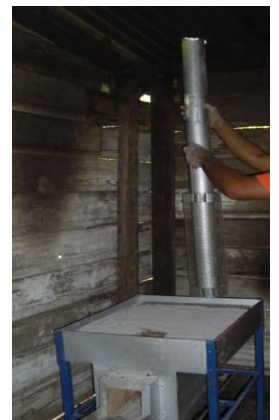
Installing (portable) improved stove
